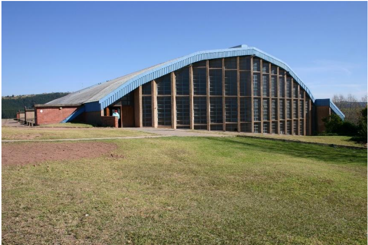
Figure 20. This big hall shortly after we finished building it.
