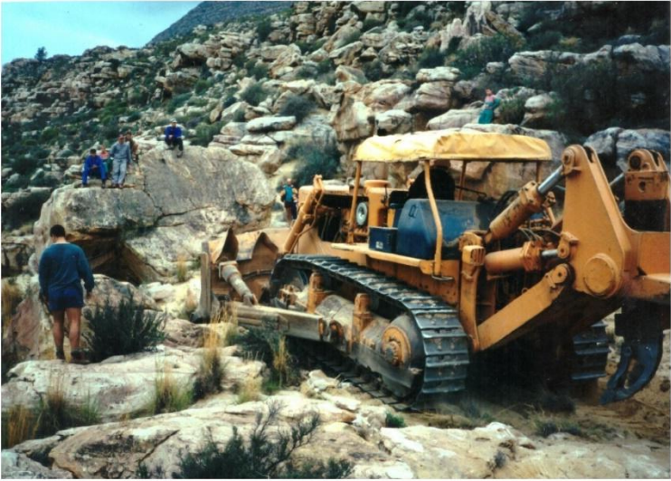
Figure 48. Building the road to the house.
