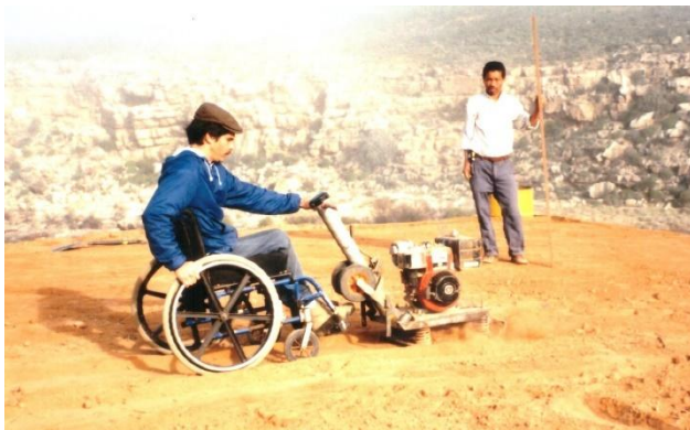
Figure 51. Japie Vermeulen compacting the soil for the main house.
