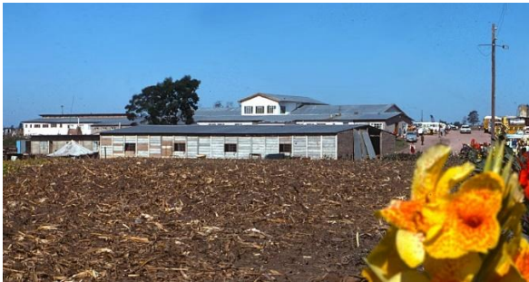
Figure 16. KSB in 1978. Between Erlo's house and the workshop.
